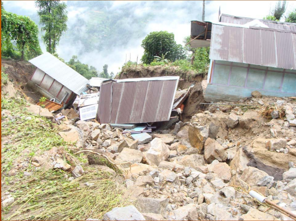
DAMAGES TO NANDOK VILLAGE DUE TO PIPE BURST
