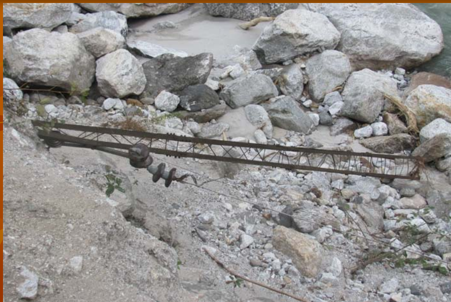
DAMAGED HIGH TENSION LINE
