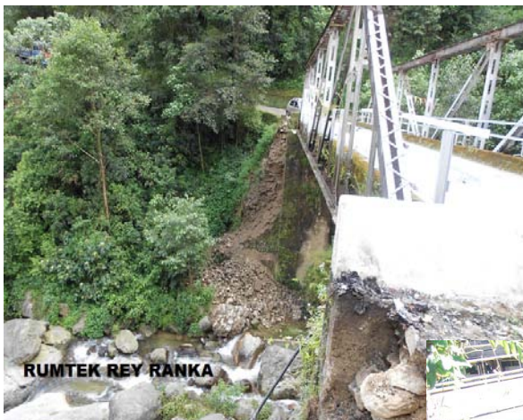
The damaged wing walls along the approaches.
