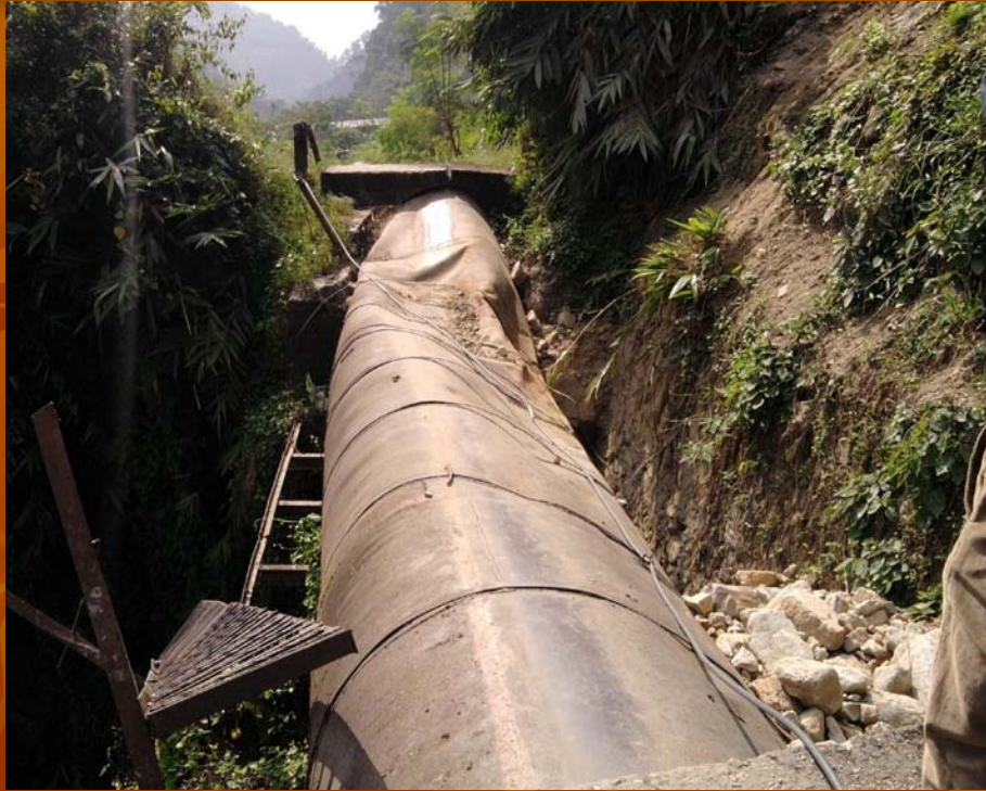
DAMAGED WATER CONDUCTOR
