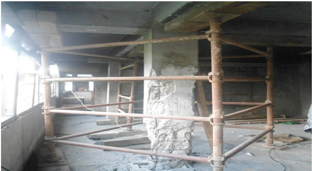
Temporary propping support to a damaged building in Gangtok
